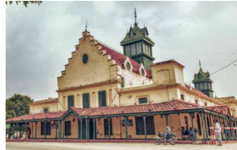
Tollington Building (City Heritage Museum), Mall Road, Lahore
